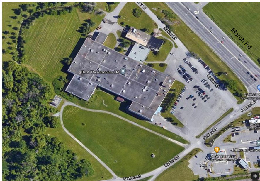
Figure 3-3: Aerial view of the Best Theratronics Ltd. Facility (Source: Google Maps)
